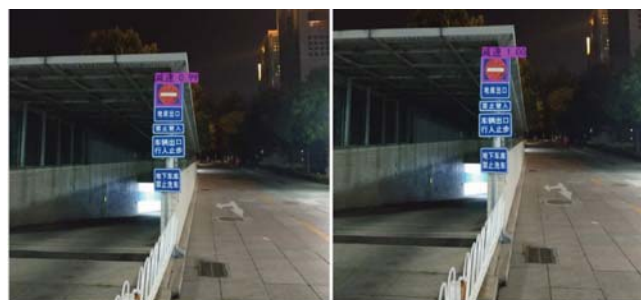
Fig. 8 before and after improvement (Night)
